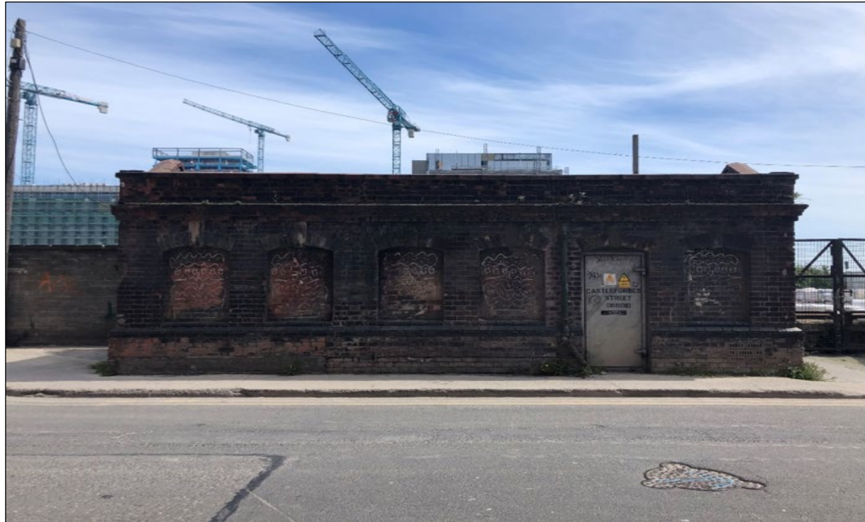
Figure 2.7: Detached single storey electricity substations external to the site on Castleforbes Road. Source: TPA, May 2020.
