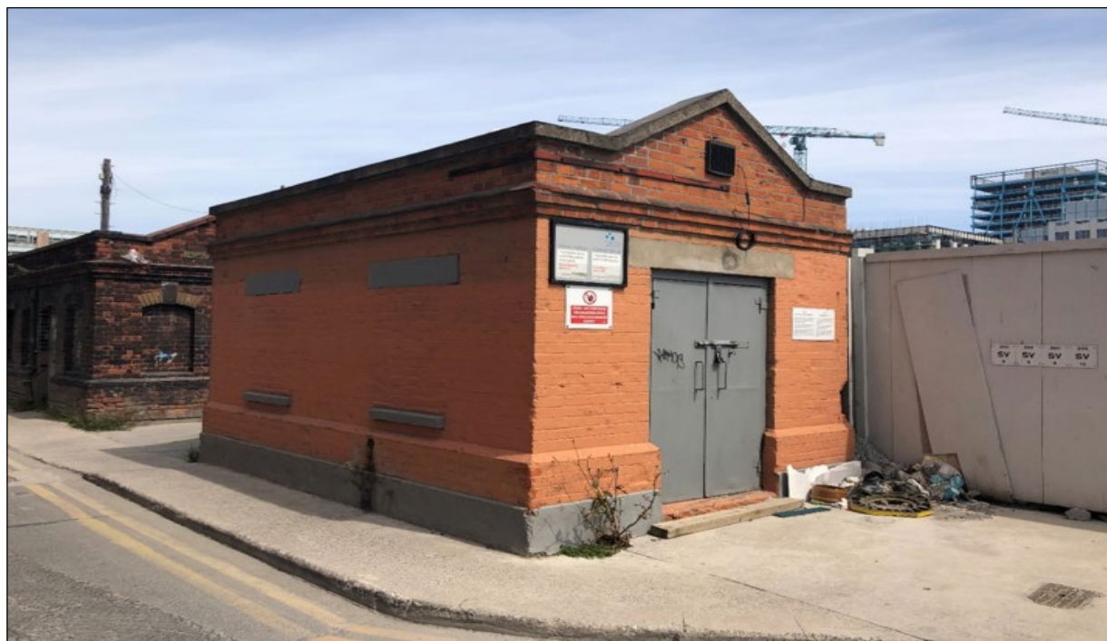
Figure 2.8: Detached single storey electricity substations external to the site on Castleforbes Road. Source: TPA, May 2020.
