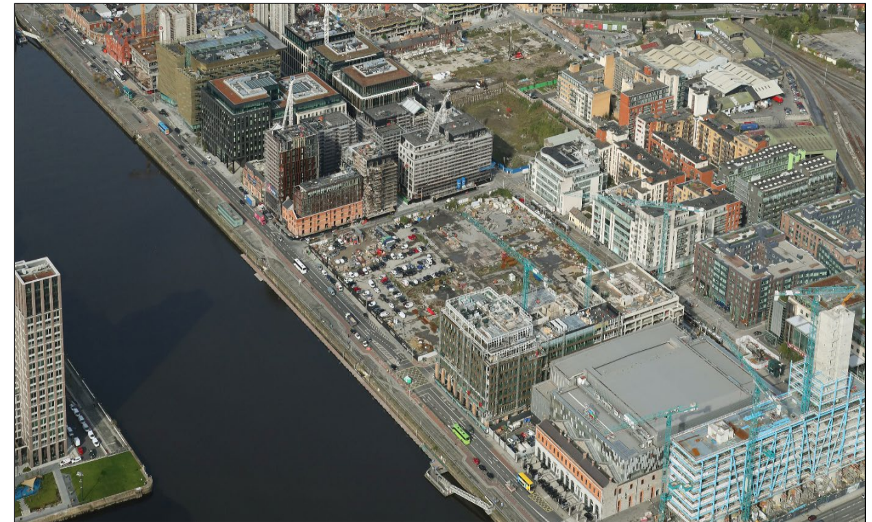
Figure 1.4: An aerial view, taken in November 2019 illustrates the scale of the site in an urban context. Source: Barrow Cookley, November 2019.
